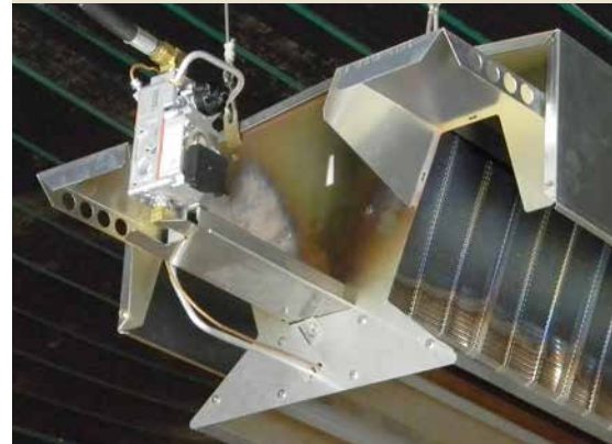
Low-Pressure, Zone Control Model permits 12 V DC battery back-up.
