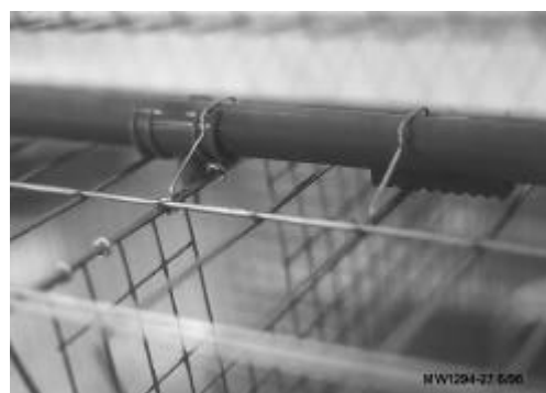
Figure 8. Wire Clip Installation
