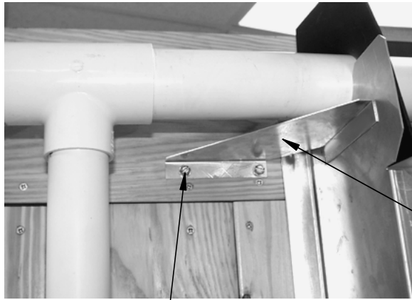
Figure 15. End Panel Support Installation
